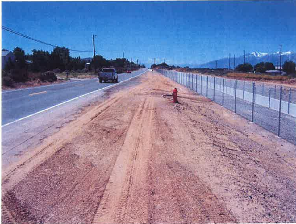
South Edmonds Drive looking south from Valley View Drive
