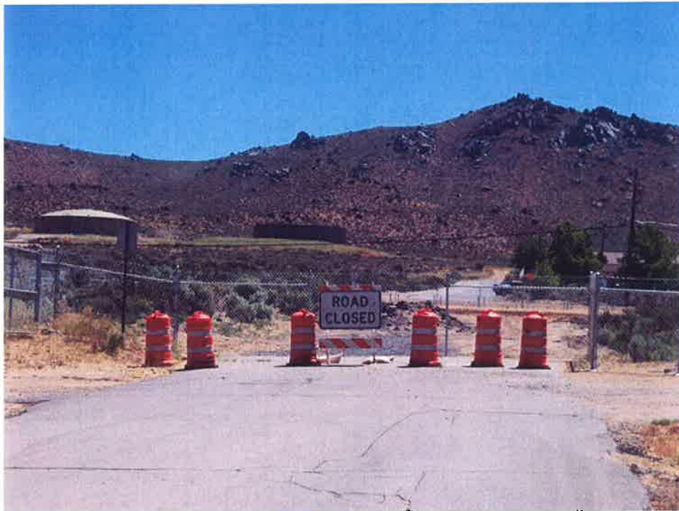
Valley View Drive dead end looking east towards Prison Hill.
