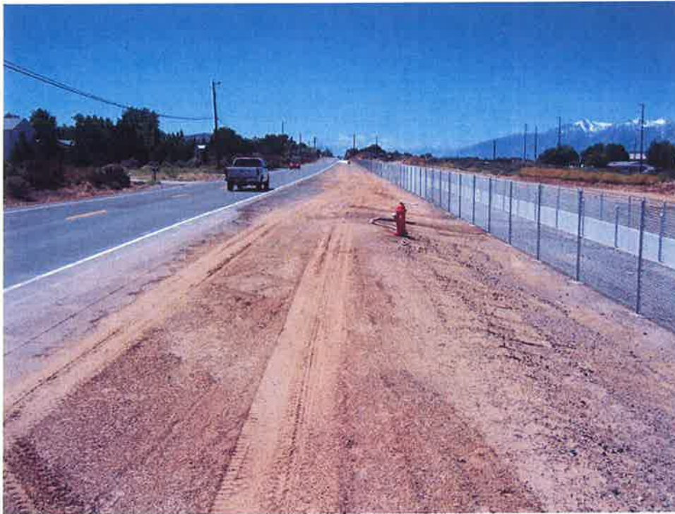
South Edmonds Drive looking south from Valley View Drive
