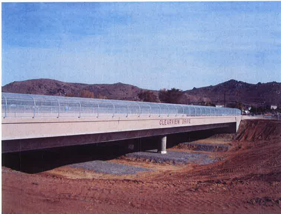
Clearview Drive Bridge
