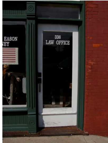
WOOD TRIM at DOORS, WINDOWS and BASE OF SIDING at COMMERCIAL STOREFRONT REINFORCES TRIM DESIGN
