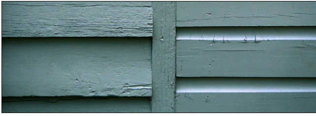
The original building to the left has clapboard siding, and the later addition, located to the right, has German siding.
