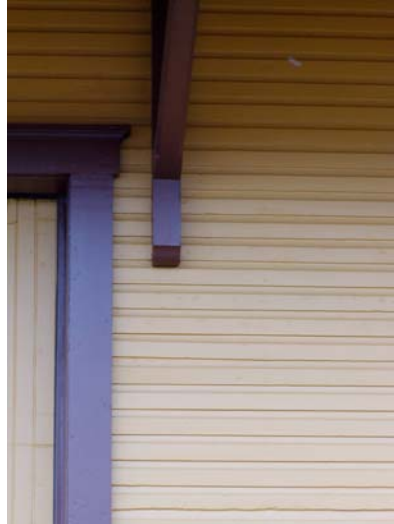
TYPICAL ‘LAPPED’ SIDING
