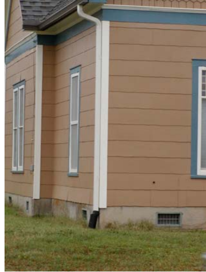
ASBESTOS SIDING which RETAINS THE WINDOW TRIM, CORNER BOARDS and FASCIA
