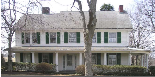
Wood clapboard siding is one of the most common historic exterior wall materials in Hopewell Township.
