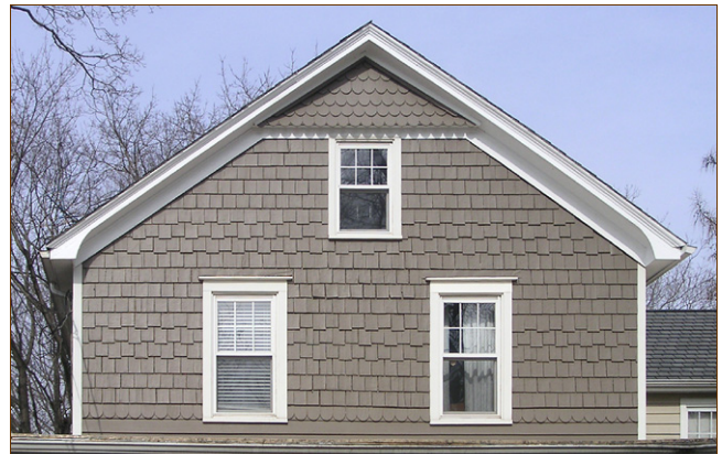
This house combines fishscale, beveled and staggered shingles.
