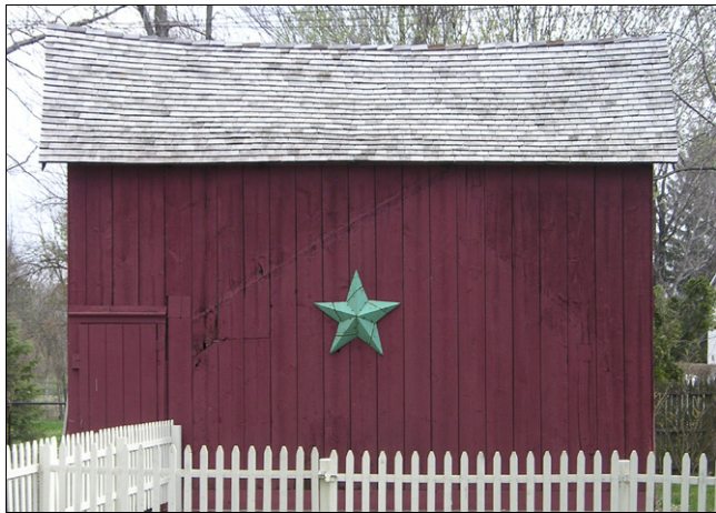
Agricultural outbuildings historically were typically painted red and usually featured vertical board or board and batten siding.
