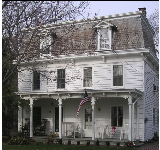
The owners of each half of this semi-detached house applied a uniform paint scheme, making it appear like a larger single home. Architectural woodwork details including the overhanging cornice, decorative brackets and porch posts remain and provide architectural richness.
