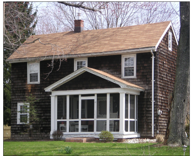
The dark brown color of these stained beveled shingles blends with the natural surroundings.
