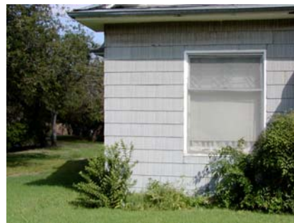
ASBESTOS SIDING with HISTORIC TRIM REMOVED
