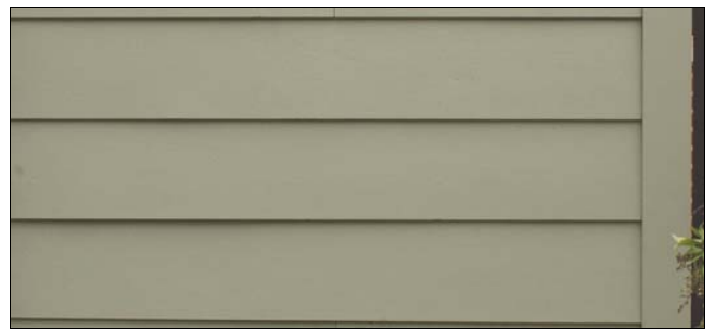
Fiber-cement siding material is a good economical alternative for an addition to an historic house. The surface of the Hardiplank siding above was painted to match the existing paint scheme.
