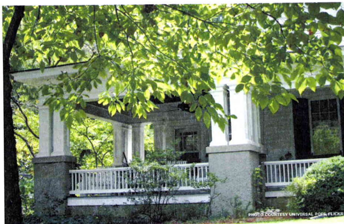
Example of a well-shaded wraparound porch on a historic home in Oxford, North Carolina.
