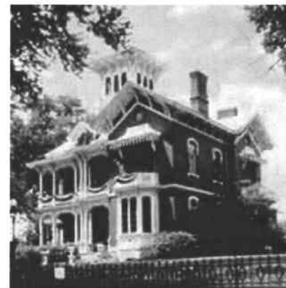
19th century buildings used porches, cupolas, and awnings to make them more comfortable in the summer. Photo: NPS files.
