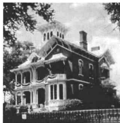
19th century buildings used porches, cupolas, and awnings to make them more comfortable in the summer. Photo: NPS files.
