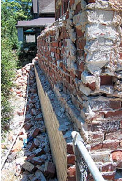
*Though the bulk of many historic brick walls are composed of common brick that is hidden from view, what we see on the exterior is a layer of veneer brick. Here peeled off the wall.*
