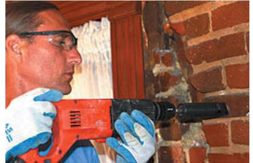
*Though the bulk of many historic brick walls are composed of common brick that is hidden from view, what we see on the exterior is a layer of veneer brick. Here peeled off the wall. Photos courtesy Nancy Snyder*
