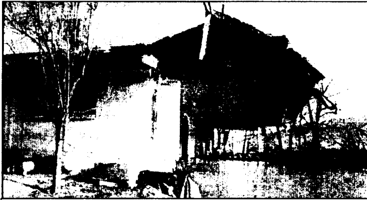
Impacts of Channel Migration on a House in Dayton during the 1977 Flood Event. (Photo courtesy of the Reno-Gazette Journal)
