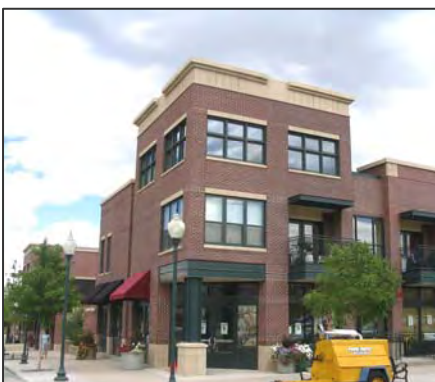
The City will seek to expand its housing variety—encouraging the incorporation of a wider range of attached living options, such as these fourplexes (top) and lofts (bottom).
