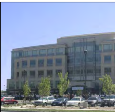
Downtown revitalization activities should build upon opportunities created by the City's state government cluster.
