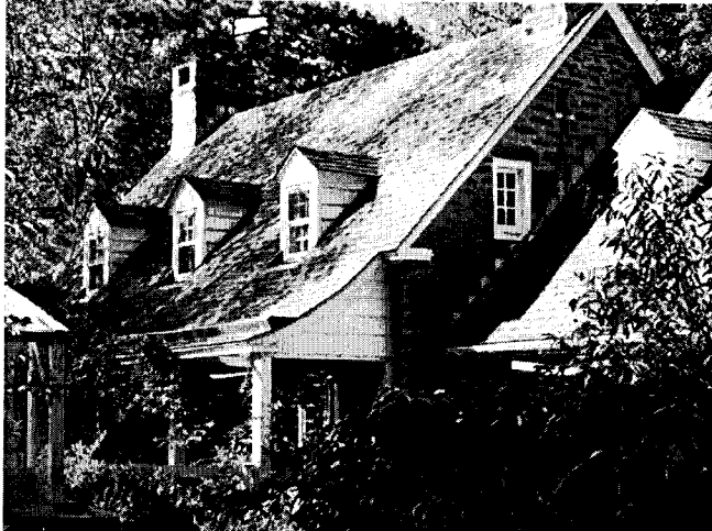
Note the extensive surrounding trees, deep porch, and masonry walls. These elements assist in keeping historic houses cooler in summer months.
