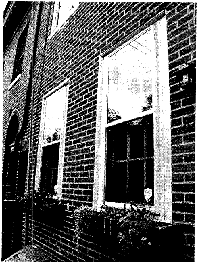
Using exterior storm windows is an effective method for reducing exterior energy losses in historic buildings.
