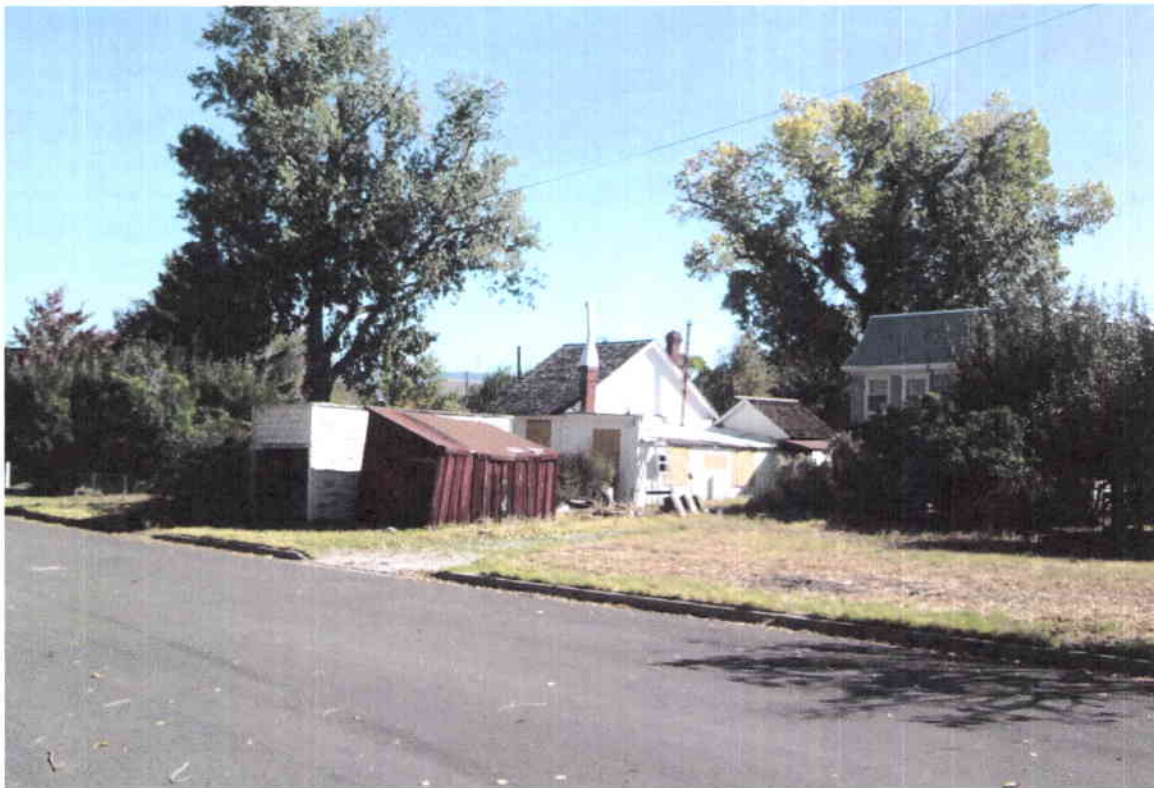
View from Ann St. looking S.E. across property toward existing structures
