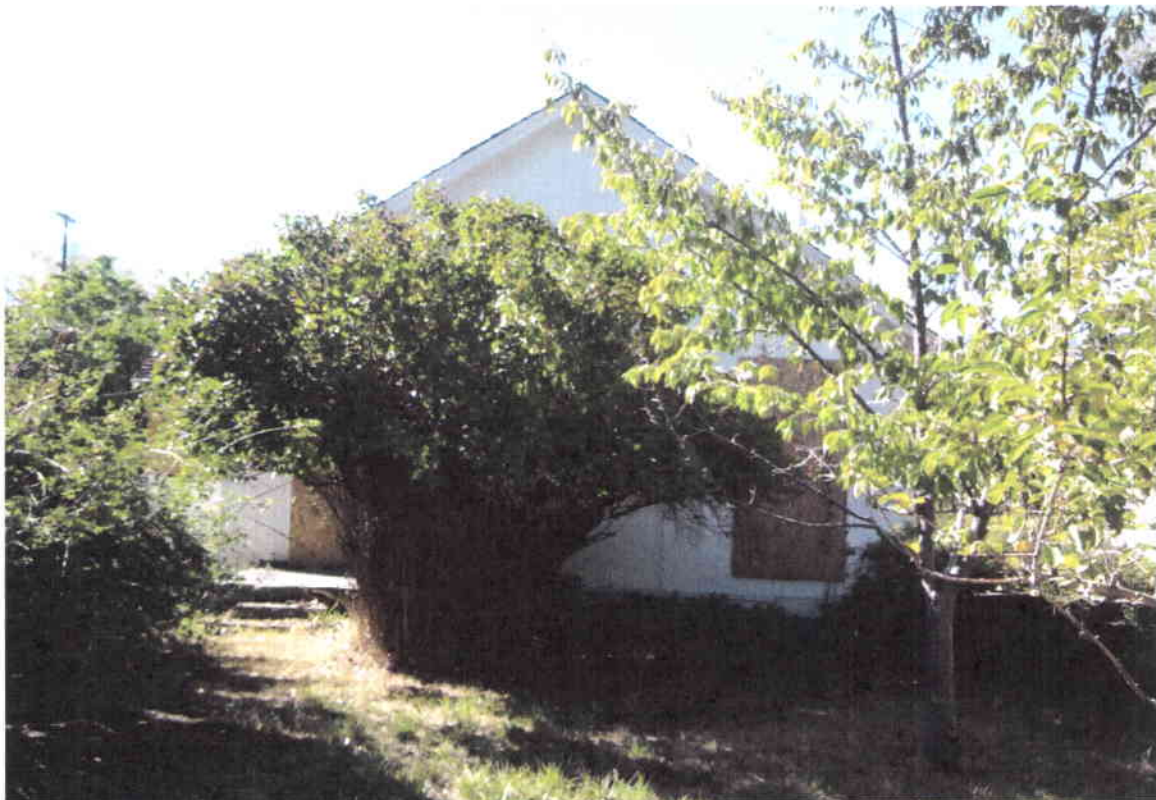
View from Division St. looking West at existing residence
