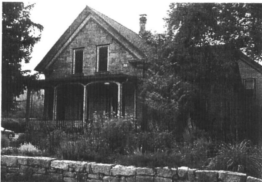
TOP: No fewer than three bay windows adorn the 1875 Olcovich-Meyers House, designed in a late Italianate style with Gothic Revival gables. ABOVE: The warm-toned local sandstone is used in major public buildings and in a few houses, including the circa 1883 Edwards House, where it was laid in a random ashlar pattern.
