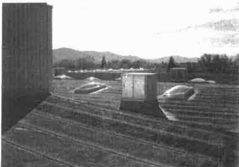
Overall view of Upper roof section
