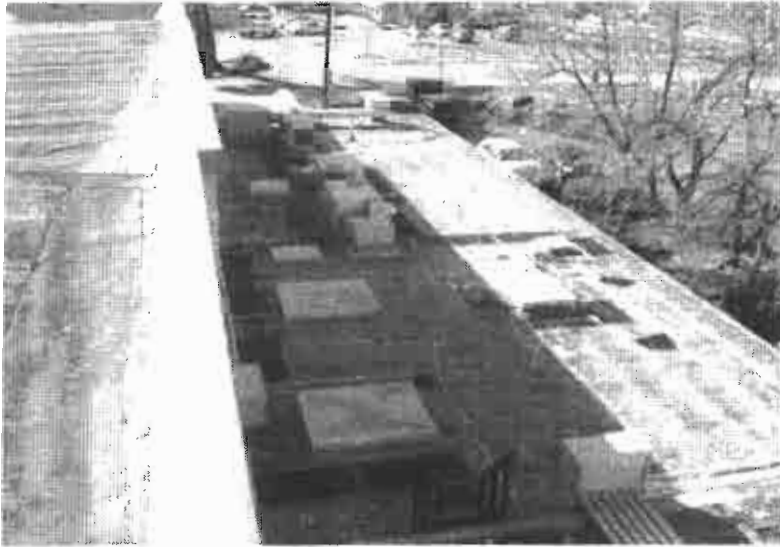
View of lower roof section
