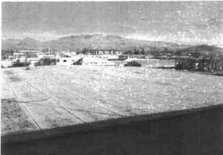
Overall view of upper section of roof system
