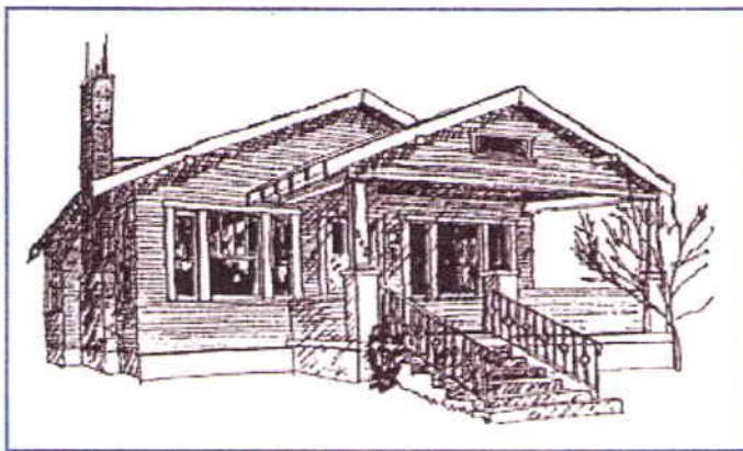
The Craftsman Bungalow was the dominant residential building style in the United States between 1905 and 1920. The house at 202 North Curry Street, illustrated above, is a typical example. Note the exposed rafter ends, the purlins decorating the gable end, the 3 part windows with four-lights-over-one-light and the typical front porch with typical elephantine posts on piers. Also, 502 West Spear Street is an excellent example of a brick Bungalow and is similar to the brick Bungalows prevalent in southwest Reno. Few examples of the style survive in Carson City.
