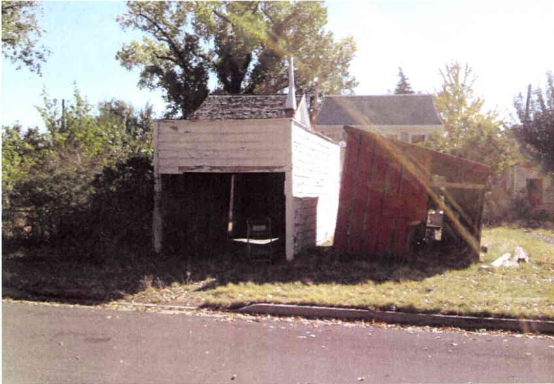
View from Ann St. looking at existing Carriage House & Shed
