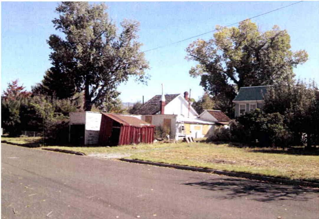
View from Ann St. looking S.E. across property toward existing structures
