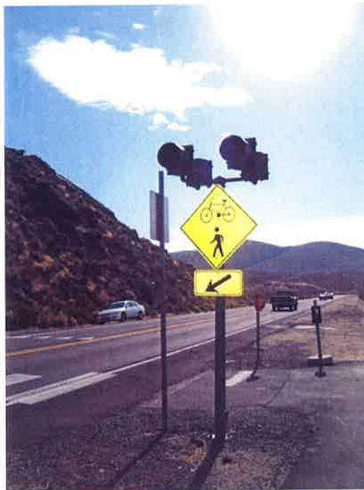
Flashing Pedestrian Crossing Indicators
