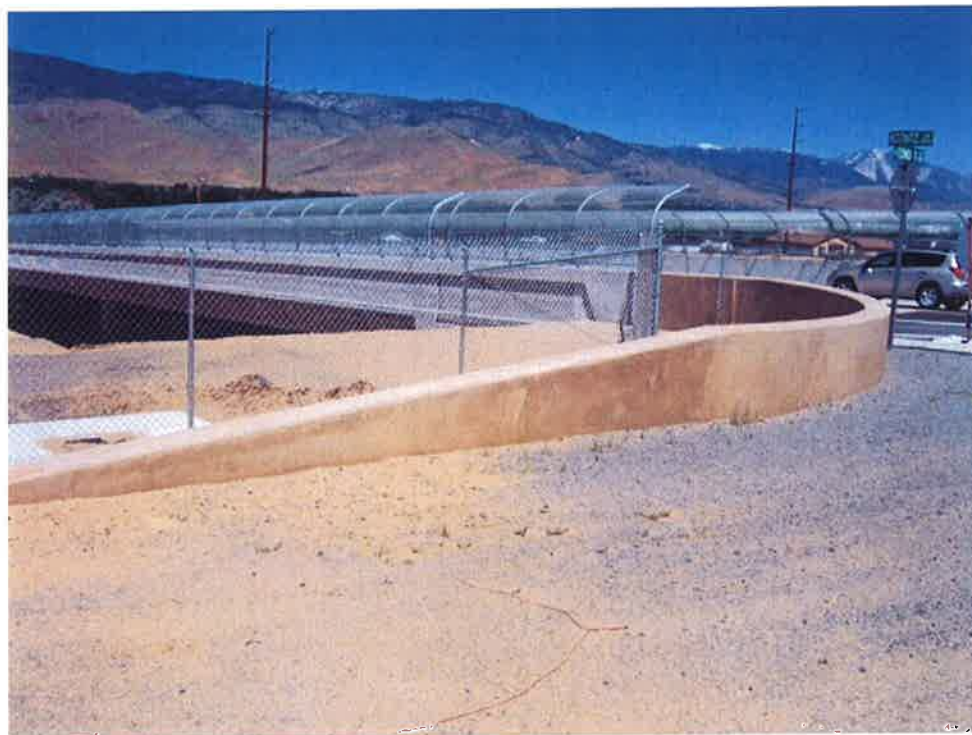
Koontz Lane bridge concrete barrier rail transition.
