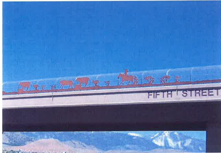
Fifth Street Bridge – The Ranching Theme
