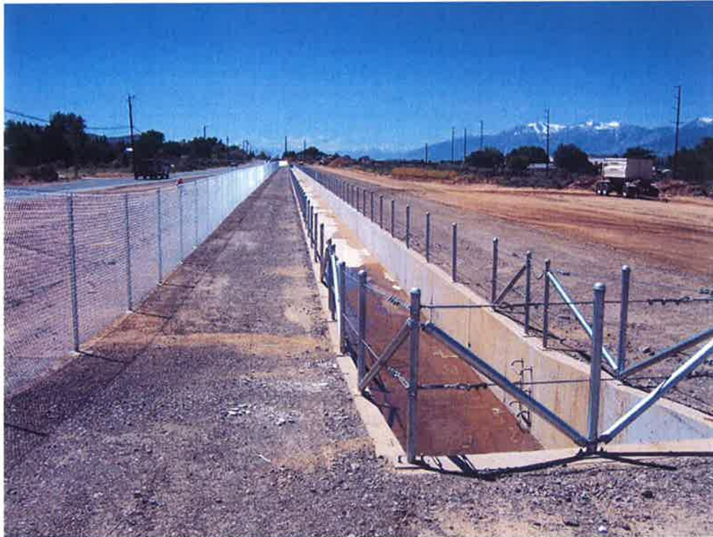
NDOT concrete drainage channel
