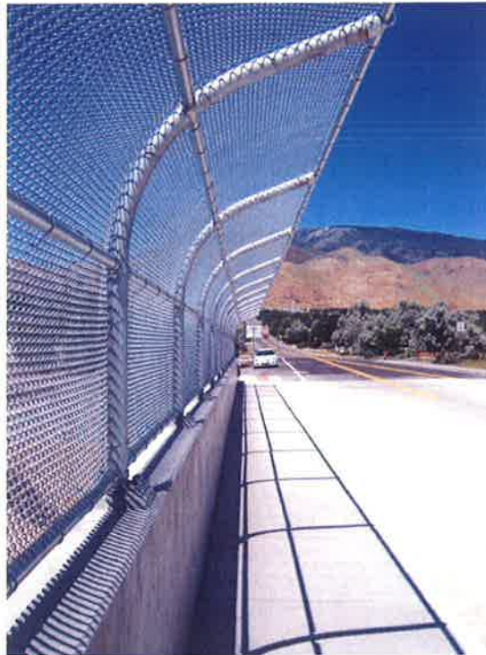
Railing on Koontz Lane Bridge
