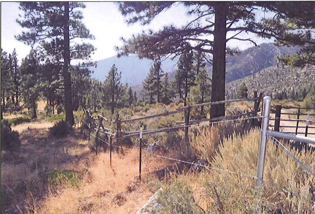
Photo – At the upper gated entrance, a new three-strand barbed wire fence extends to the south.
