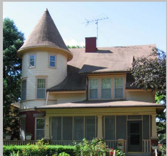
If enclosing a porch, using large single pane windows or single panels of screening are most appropriate, especially when the original porch framework is left exposed. This treatment maintains the illusion that the porch is still an open space.
