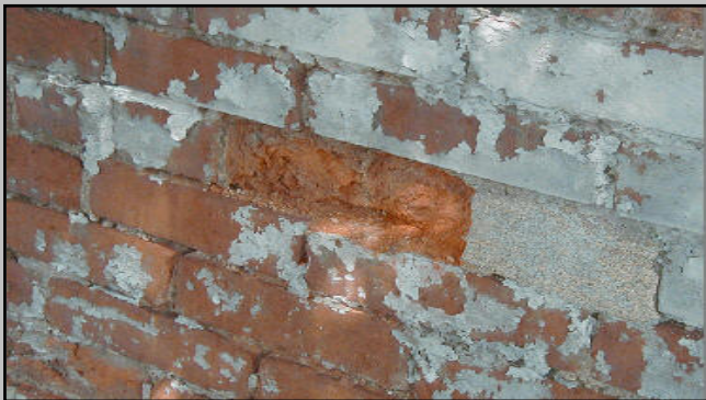
Never sandblast or use high-pressure power washing to clean masonry. Doing so can compromise the building structure by scarring masonry surfaces beyond repair, which will allow excessive moisture into the masonry.
