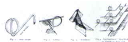
Folsom Snow Guard Company of Boston, Massachusetts advertised three models of snow guards in the 1906 Sweet's Indexed Catalogue of Building Construction . [click image for larger view]
