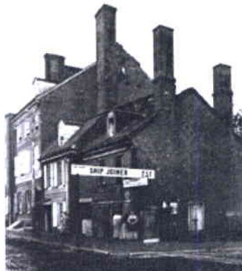
The pole gutters on the roof at 757 Swanson Street, Philadelphia in 1868 divert rainwater to a short cylindrical downspout. Moisture damage is evident on the wall of the building below the end of the pipe where there is no downspout extension. (Print & Picture Collection, The Free Library of Philadelphia) [click image for larger view]
