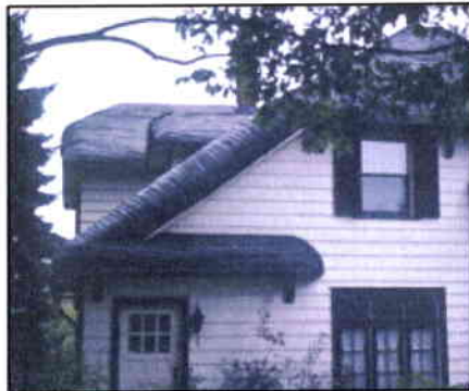
The wood shingles on the roof of this Tudor Revival house (left) were steamed and bent to resemble thatching. To aid architects and contractors to lay such special effects shingles properly, manufacturers like the Creco-Dipt Company, Inc. of North Tonawanda, New York, published roof details, like those in the 1923 Sweet's Architectural Catalogue (below). (Photograph courtesy of NPS; "Country Cottage Roof".) [click image for larger view]
