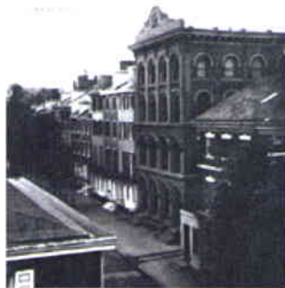
An 1871 photograph of the corner of 3rd Street, south of Walnut in Philadelphia shows a number of rain water conductor systems. In the lower left corner is a metal roof with a built-in gutter lined with metal; on the far right is a building with a wood shingle roof and a built-in gutter with exposed downspout; and in the center is a four story brick building with built-in gutters and internal downspouts. (Print & Picture Collection, The Free Library of Philadelphia) [click image for larger view]
