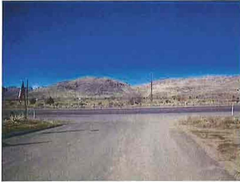
A VIEW LOOKING NORTHERLY ALONG THE SUBJECT'S EAST ACCESS POINT FROM HIGHWAY 50
