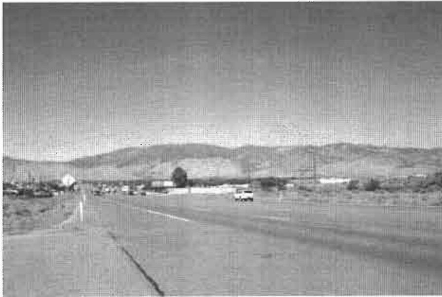
VIEW LOOKING WESTERLY ALONG HIGHWAY 50 EAST IN THE VICINITY OF THE SUBJECT
