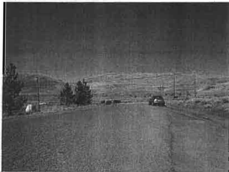
A VIEW LOOKING NORTHERLY ALONG ASPHALT DRIVE IN THE VICINITY OF THE SUBJECT
