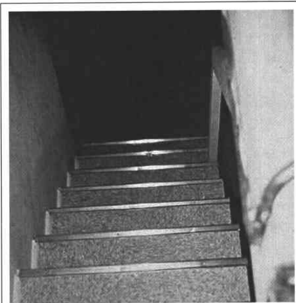
FIGURE 18.6 Enclosure of stairs in this manner is generally not appropriate in a historic property.
