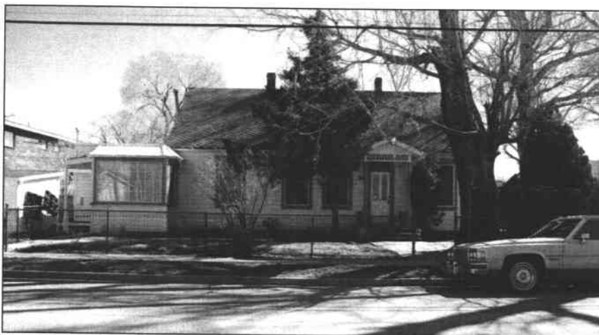
Front (west) facade
