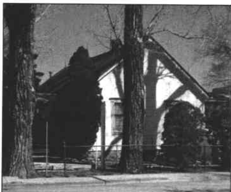
Side (south) facade
