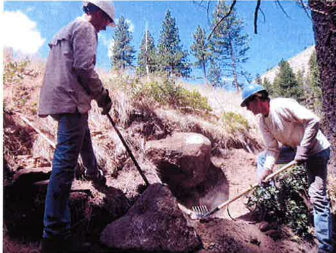
Trail under construction, south side
