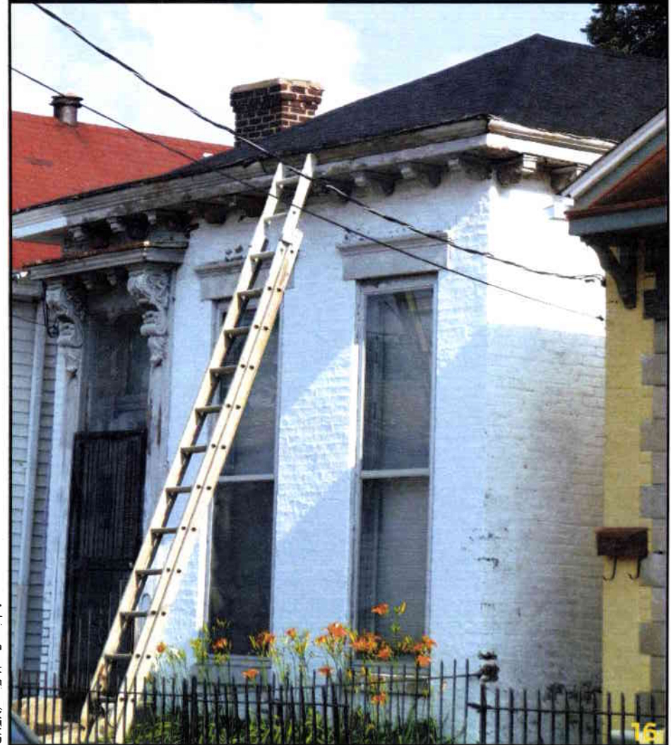
Shotgun house with hip roof and asphalt shingles Louisville, Kentucky
