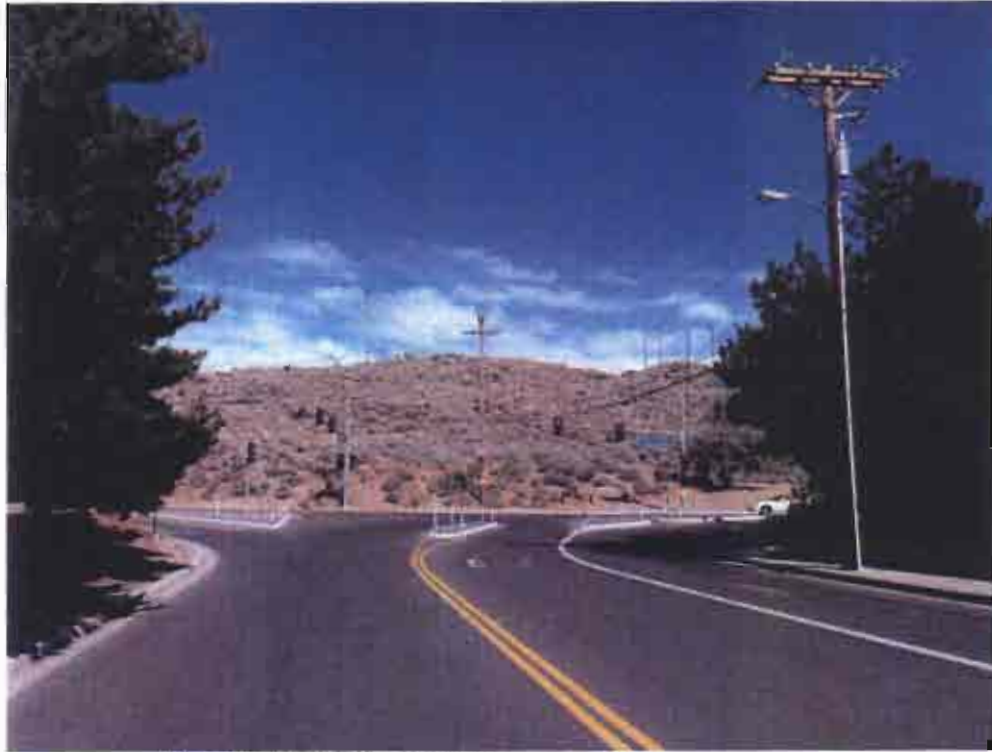
View looking east toward the site from W. Winnie Lane
