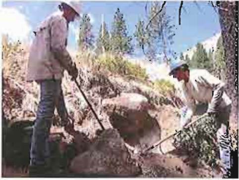
Trail under construction, south side
