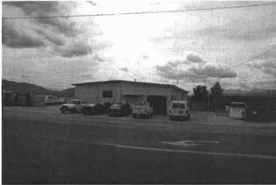
SALE IBS-5 1749 Old Hot Springs Road, Carson City
