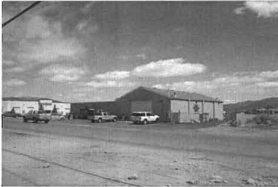
A VIEW LOOKING NORTHEASTERLY TOWARD THE SUBJECT FROM SOUTH CURRY STREET
