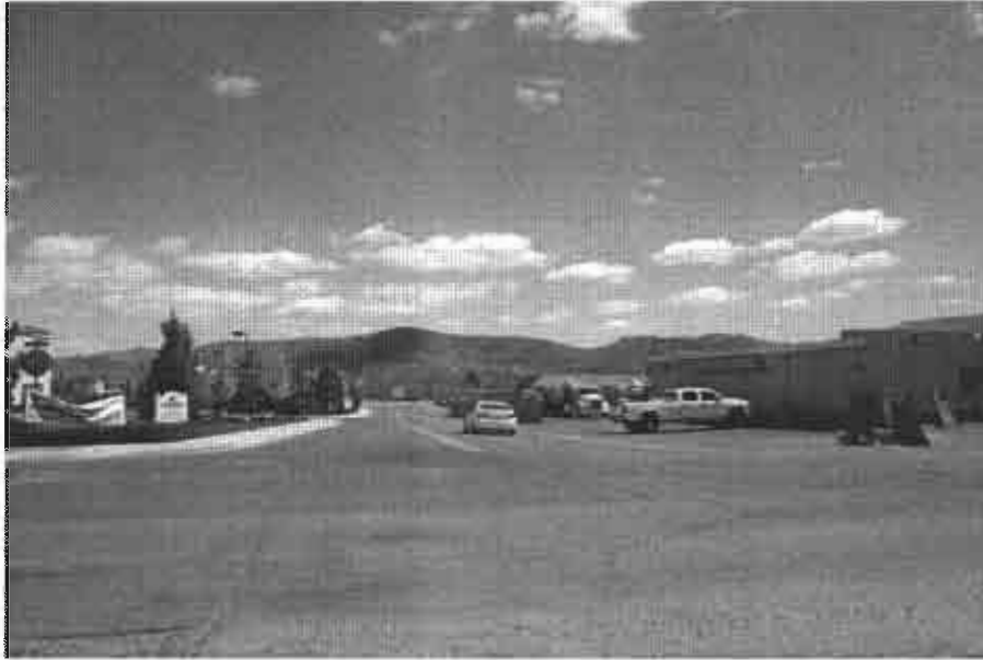
LOOKING EASTERLY ALONG RHODES STREET FROM ITS INTERSECTION WITH S. CURRY STREET
