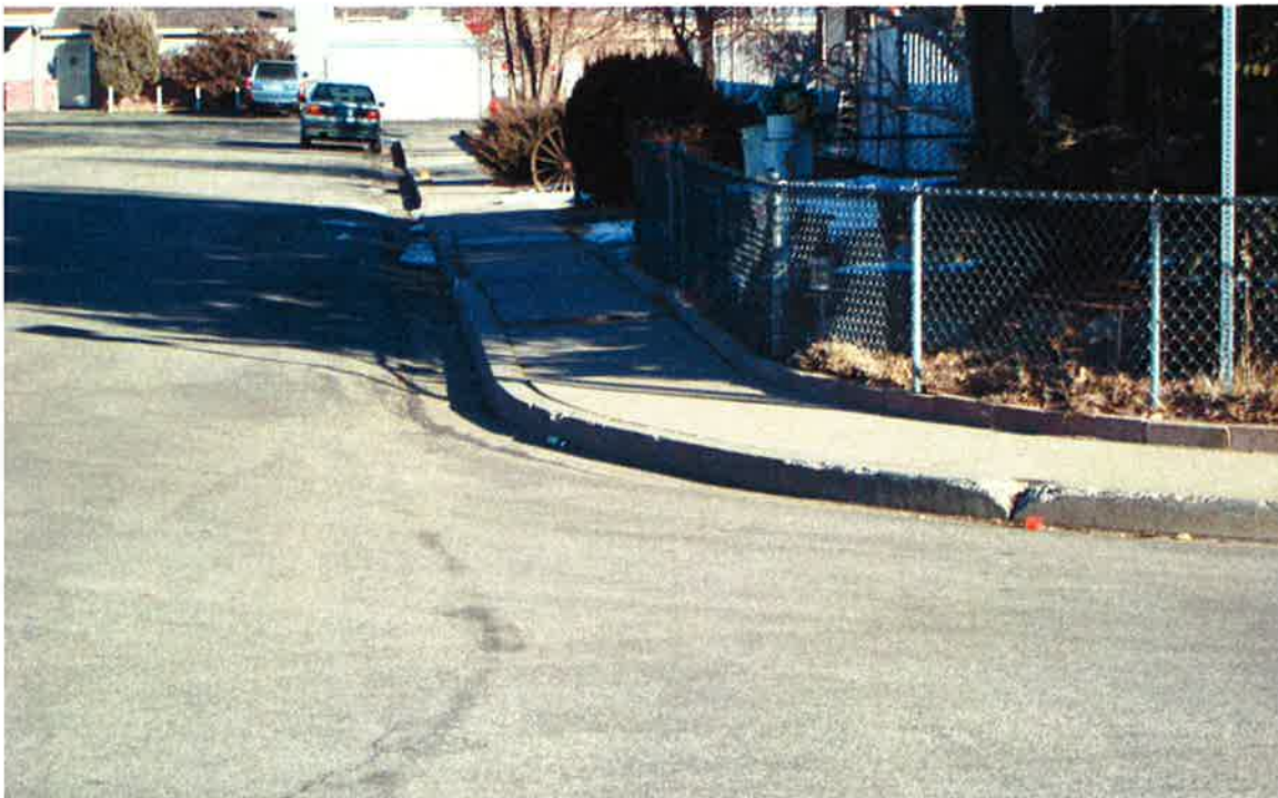
Existing Northeast Corner of Ruth St & Jerry Ln – No Curb Ramp
