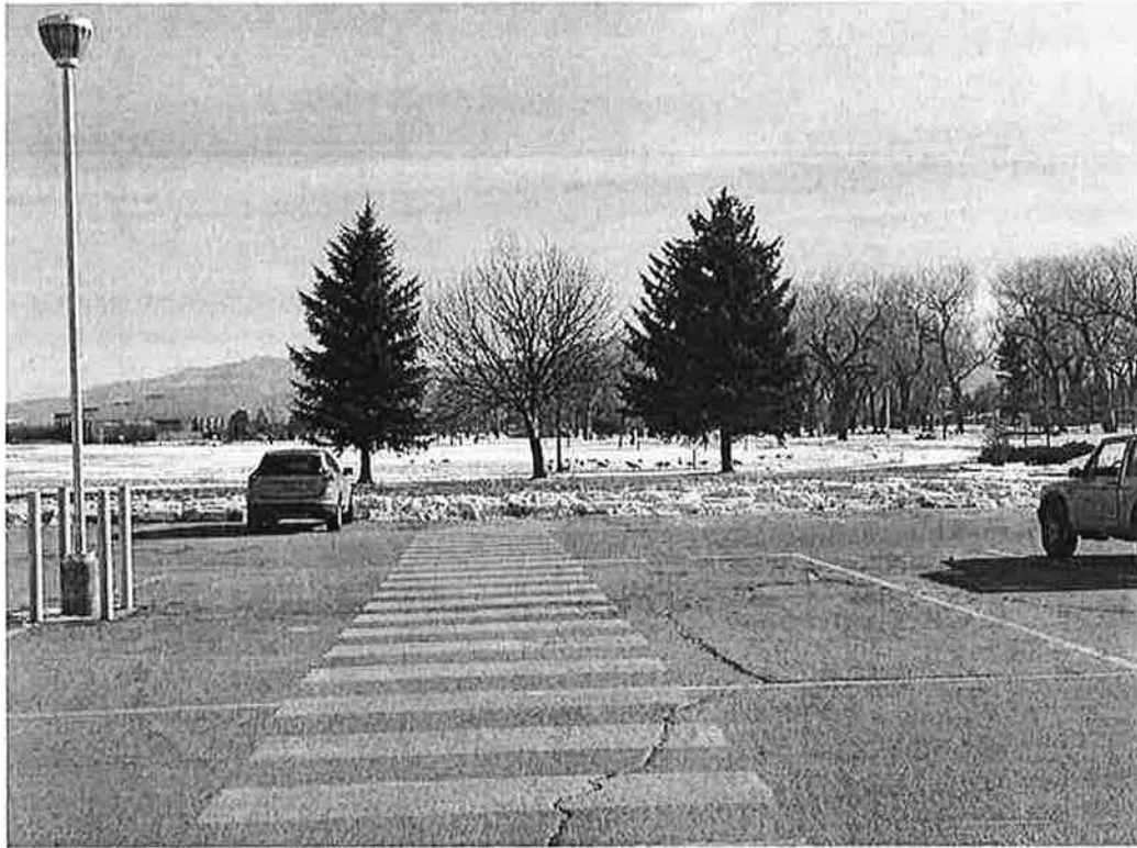
View looking east-along pedestrian corridor from Community Center Gymnasium
