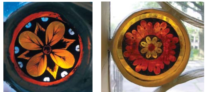
Figure 3. The entrance to the Morris-Jumel Mansion, New York City, is one of the earliest surviving installations of stained glass in the country. It features a fanlight and sidelights of large clear roundels and small bulls-eyes of red and orange glass tinted with silver stains from ca. 1810. Photo: Ken Moss.
