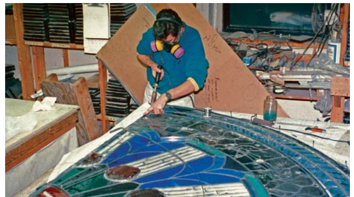
Figure 17. Total releading is very time consuming and costly and should only be undertaken when the original lead is exhausted beyond repair.
