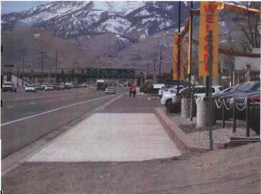
Example of Existing Concrete Path
