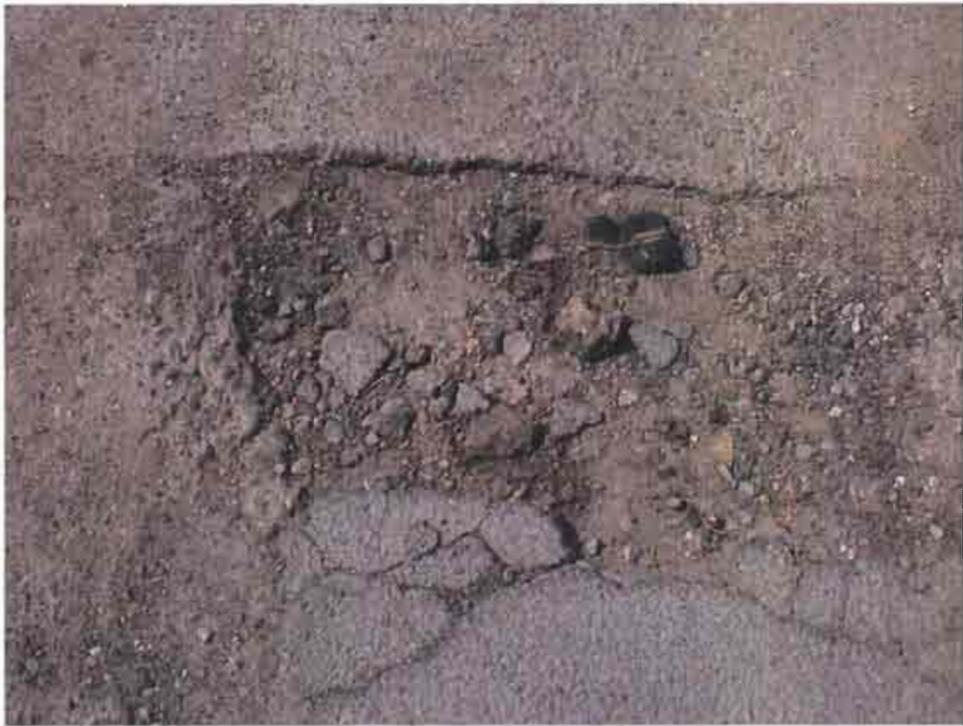
Typical Damage to Asphalt Proposed to be Replaced with Concrete
