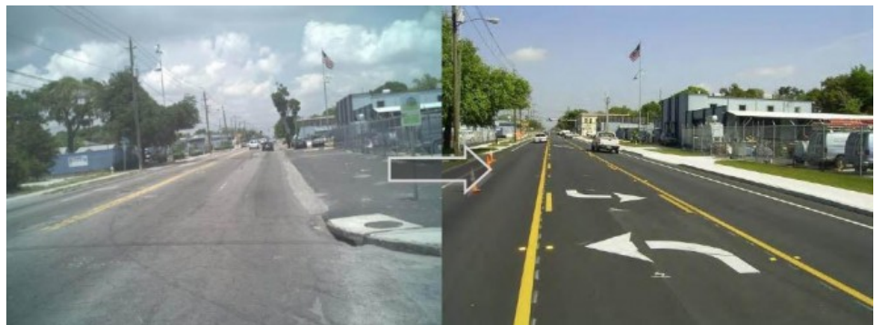
Nebraska Avenue, A Typical 4 to 3 Lane Rightsizing Project (Photo Credit: Florida DOT)
