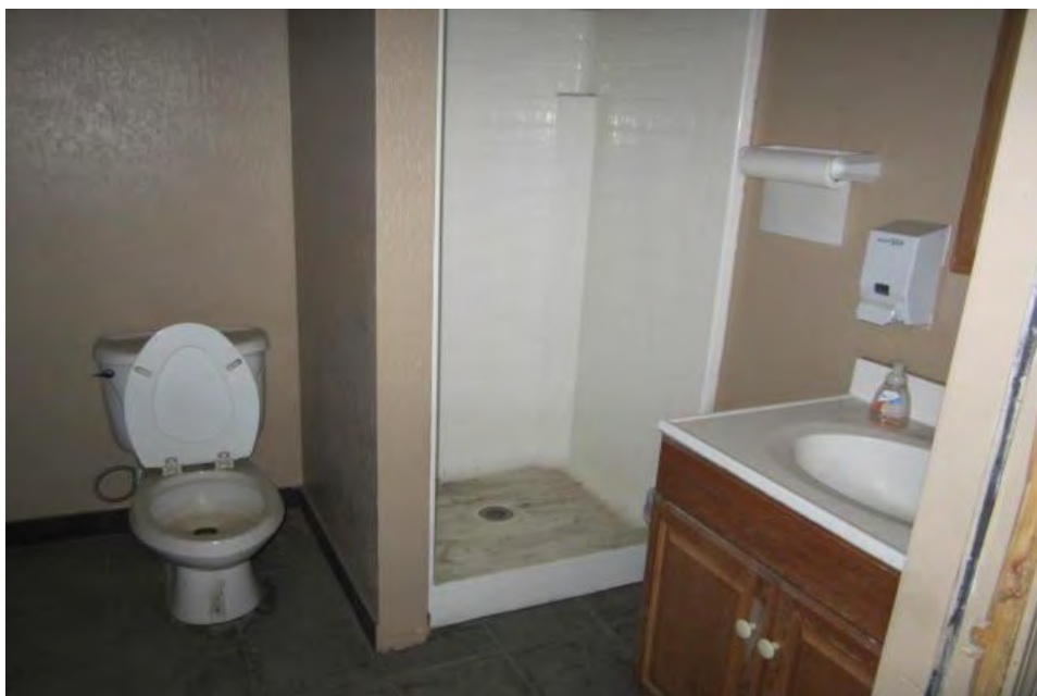
VIEW OF A TYPICAL RESTROOM IN THE SUBJECT BUILDING
