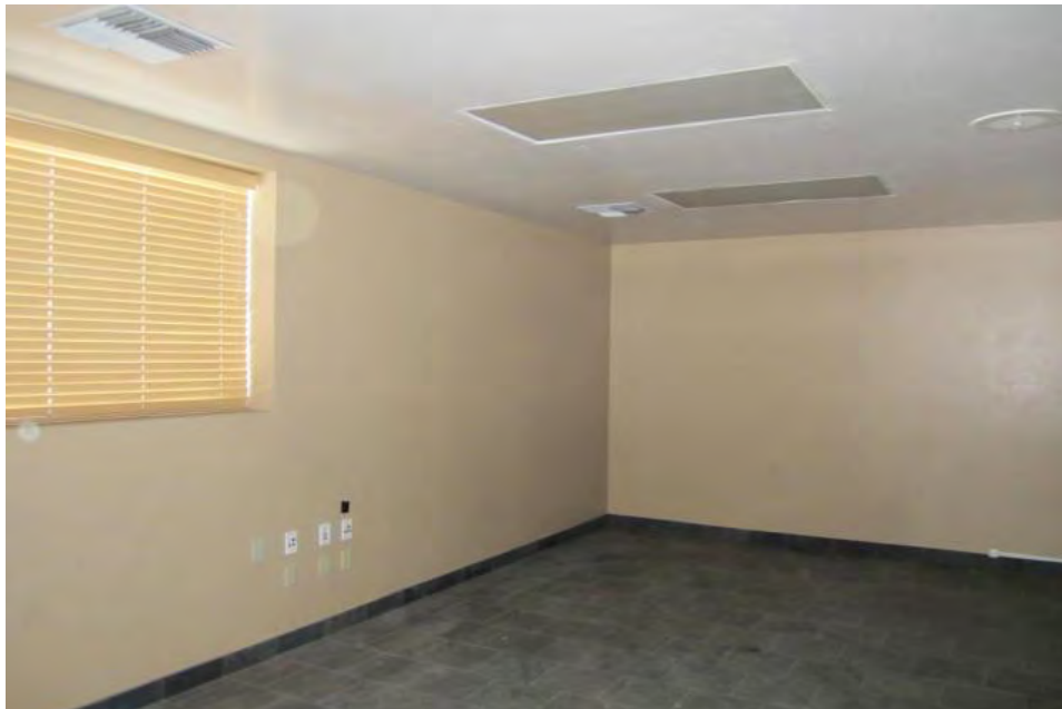
VIEW OF THE FINISHED OFFICE SPACE
