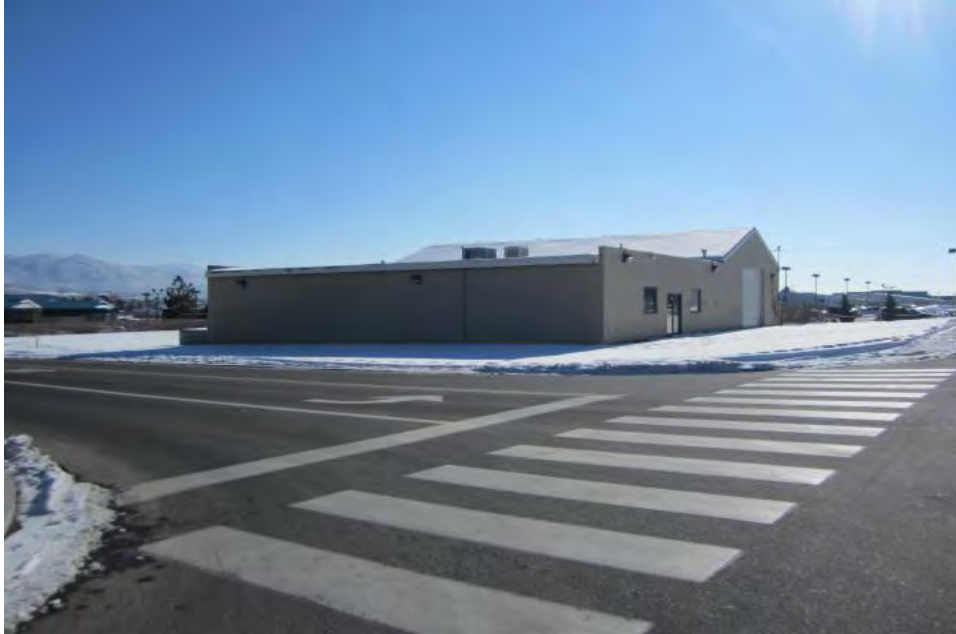
VIEW LOOKING SOUTHEASTERLY TOWARD THE SUBJECT FROM THE INTERSECTION OF SOUTH CURRY STREET AND RHODES STREET
