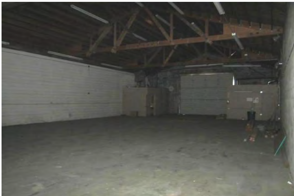
VIEW OF THE SUBJECT'S SOUTHERLY WAREHOUSE AREA
