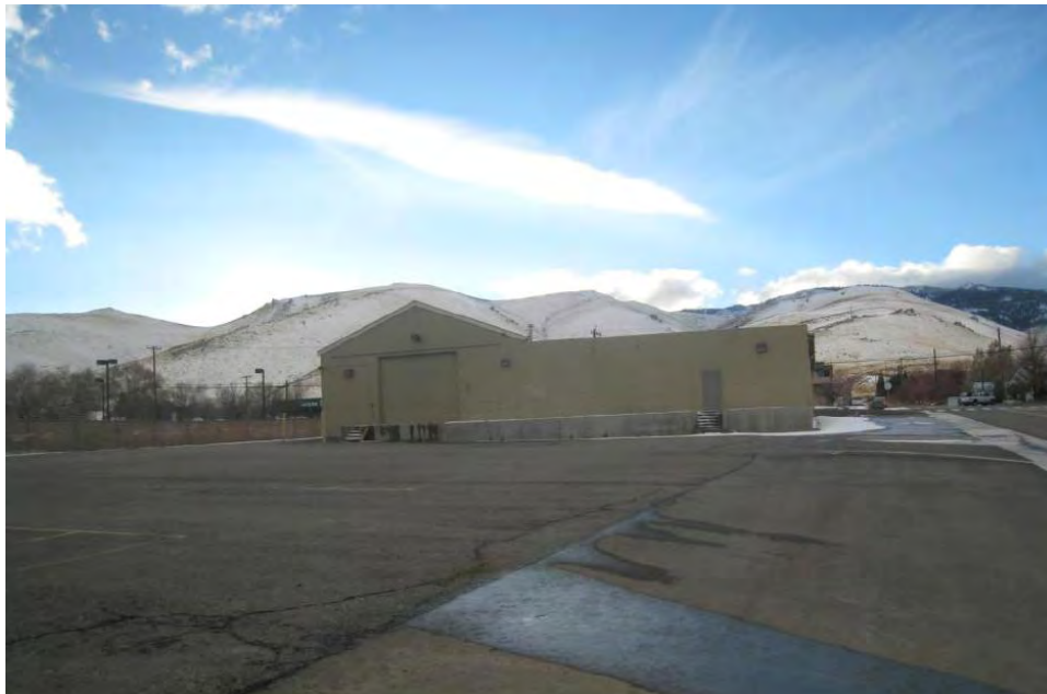
VIEW LOOKING WESTERLY TOWARD THE SUBJECT FROM NEAR RHODES STREET
