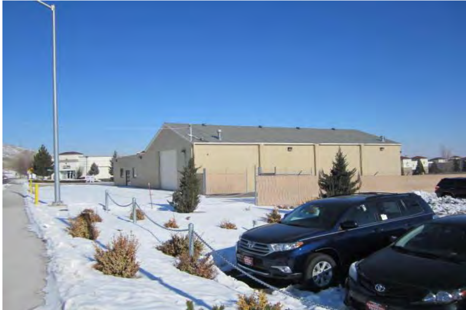
VIEW LOOKING NORTHERLY TOWARD THE SUBJECT FROM SOUTH CURRY STREET
