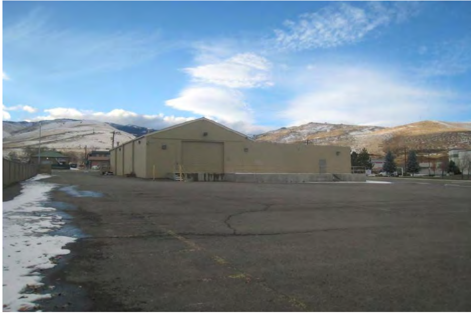
VIEW LOOKING WESTERLY TOWARD THE SUBJECT FROM ITS SOUTHEAST CORNER
