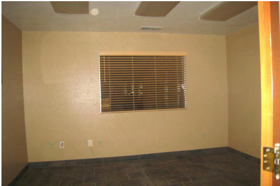
VIEW OF THE SMALLER OFFICE AREA
