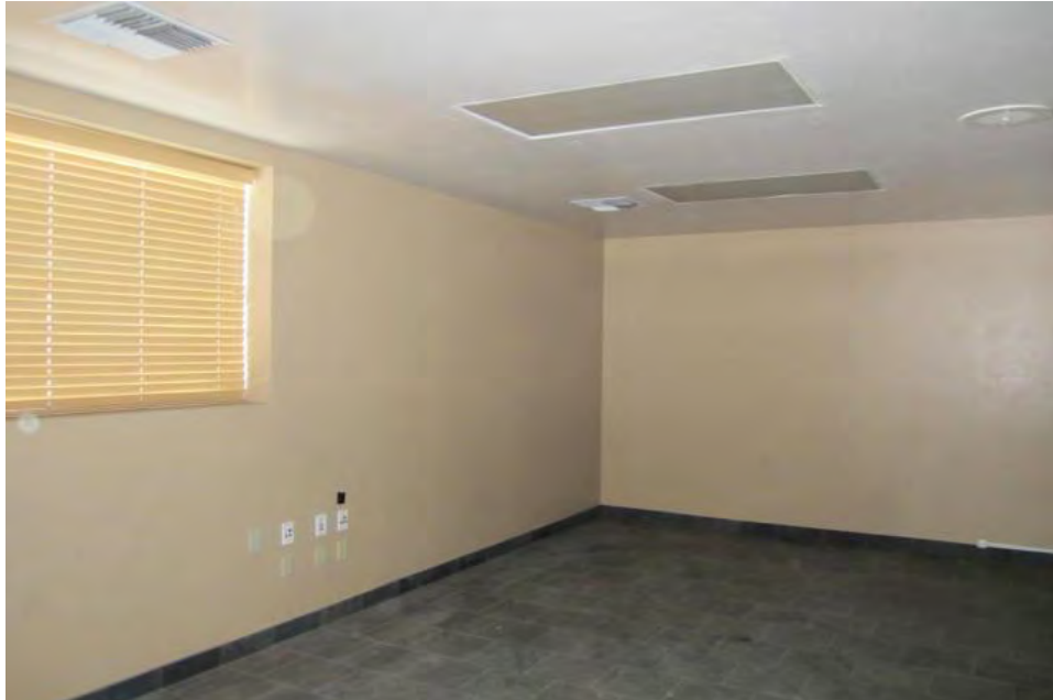
VIEW OF THE FINISHED OFFICE SPACE
