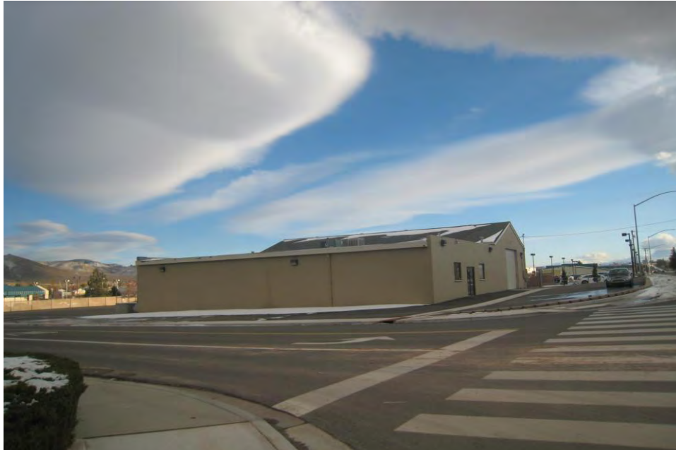
VIEW LOOKING SOUTHEASTERLY TOWARD THE SUBJECT PROPERTY FROM SOUTH CURRY STREET
