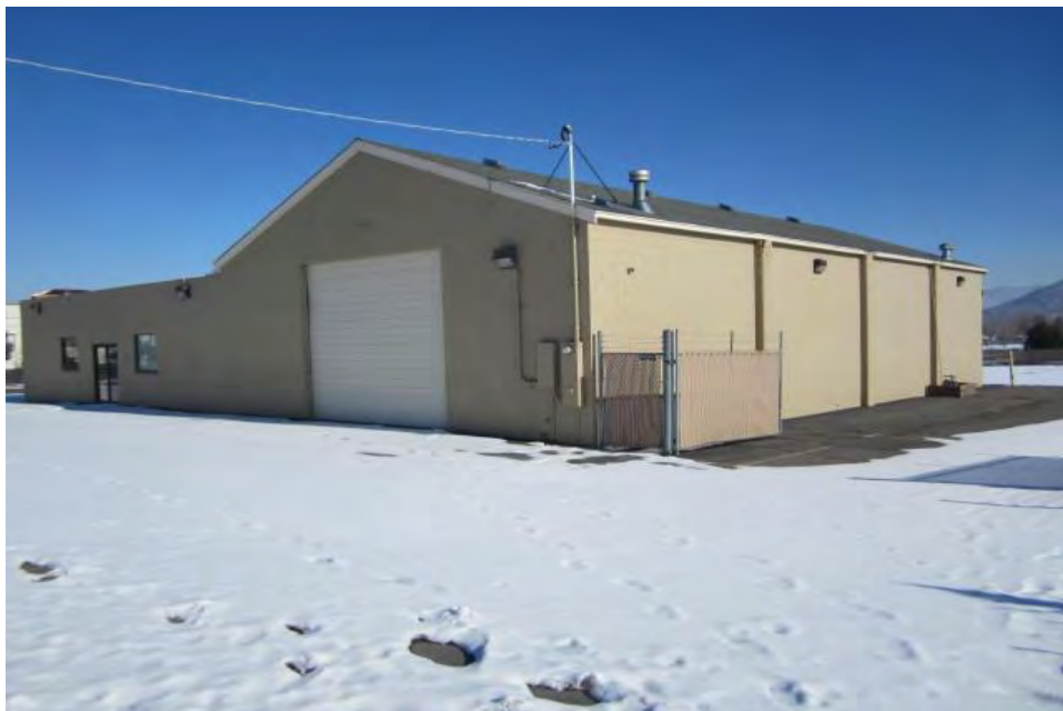
VIEW LOOKING NORTHEASTERLY TOWARD THE SUBJECT FROM SOUTH CURRY STREET
