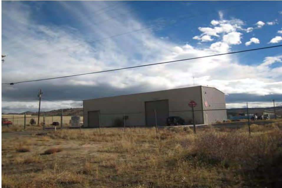
RENTAL IR-5 5835 Highway 50 East, Carson City
