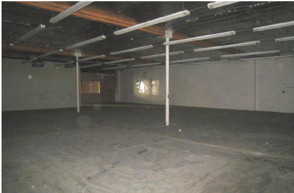
VIEW OF THE NORTH WAREHOUSE AREA
