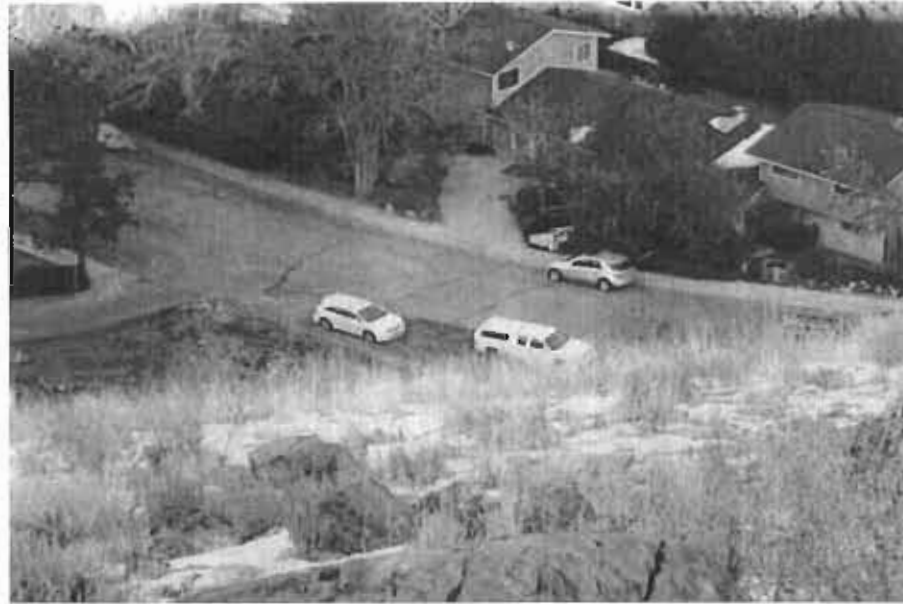
VIEW LOOKING EASTERLY TOWARD THE SUBJECT OWNERSHIP WITHIN THE SOUTH ORMSBY BOULEVARD RIGHT-OF-WAY
