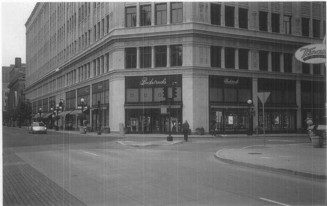
Figure 2. The Hamm Building featured fifty-six prismatic panels set directly above the awnings. Each panel contained over two hundred individual tiles. Photo shows completed project. Photo: Chad Randl
