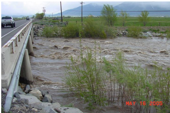
Highway 88 Bridge during 2005 spring run-off
