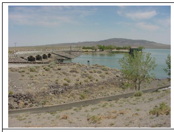
Newlands Irrigation Project Infrastructure – Churchill County, Nevada
