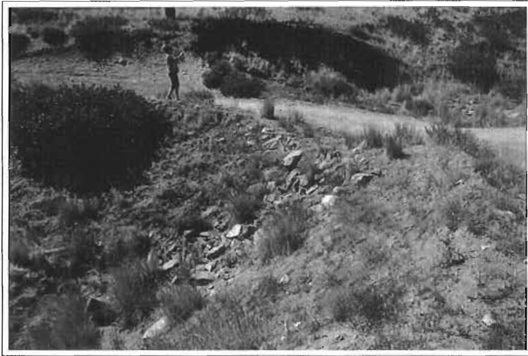
Photo 2. View of rock lined drainage near MP 1.2.
