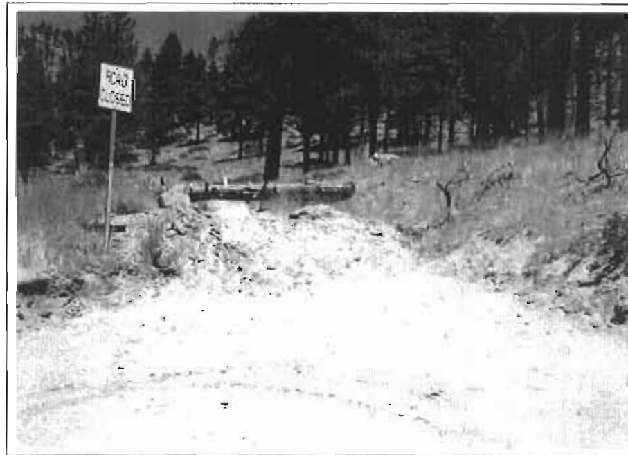
Photo 5. Road #2 closure with log, berm, and boulders near MP 1.65.
