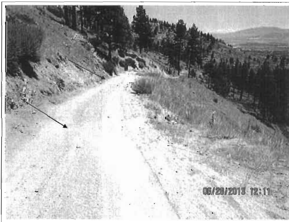
Photo 1. Rolling dips are noted by arrows near MP 2.2.
