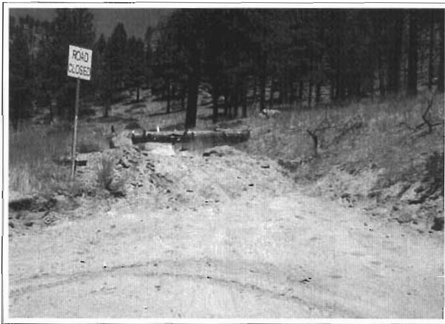
Photo 65. Road Spur #2 closure with log, berm, and boulders near mile MP 1.65. This spur terminated approximately 1200 feet into the forest near a spring.
