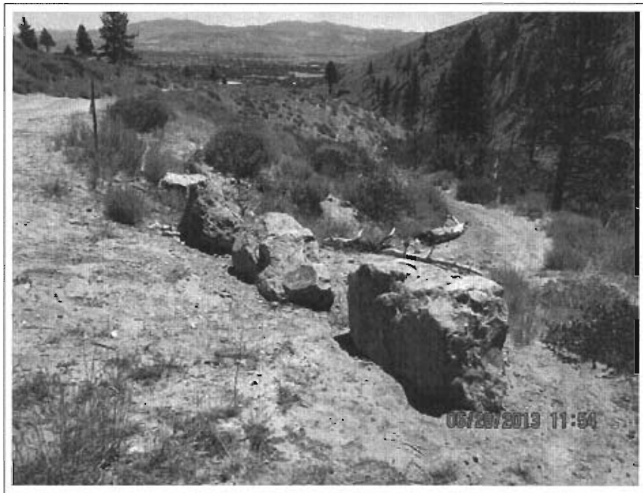
Photo 4. NDOW Road Spur closure with boulders near mile MP 1.1. This steep 540 foot long two-track spur terminated at Ash Canyon Creek and was the source of sediment in the water system. The spur had previously been used by NDOW to stock the creek with fish.
