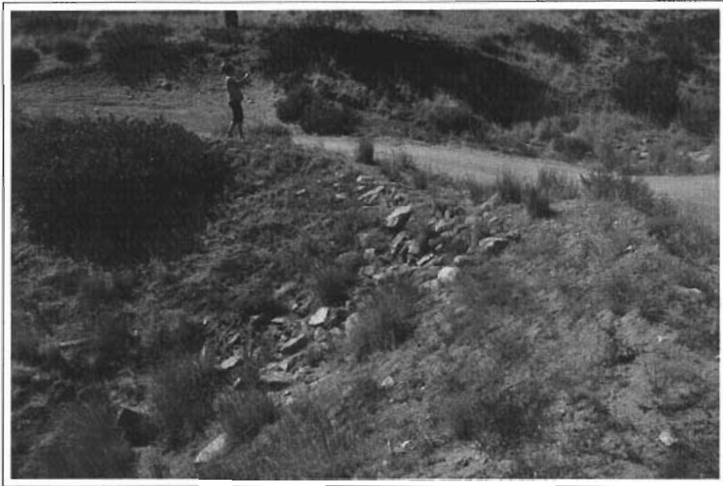
Photo 2. View of rock lined drainage near mileMP 1.2 .
