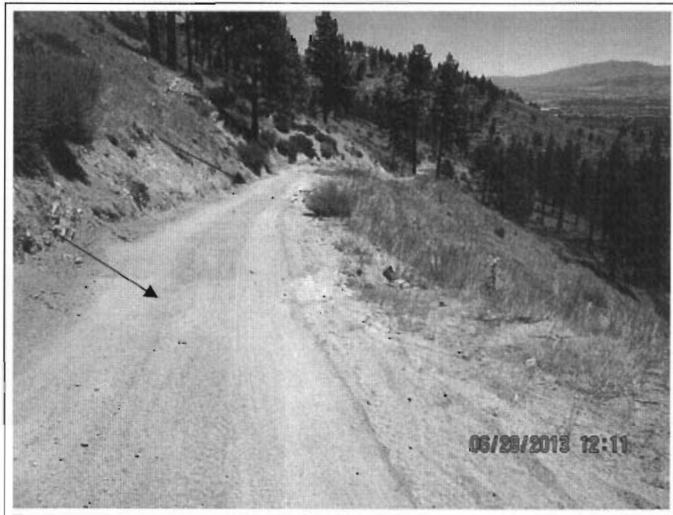
Photo 1. Rolling dips are noted by arrows near MP-mile 2.2 .
