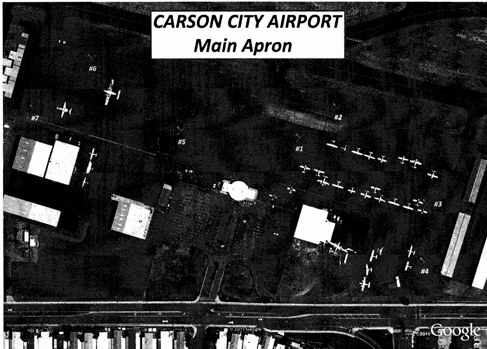
Main apron overview indicating specific areas of interest for reconstruction
