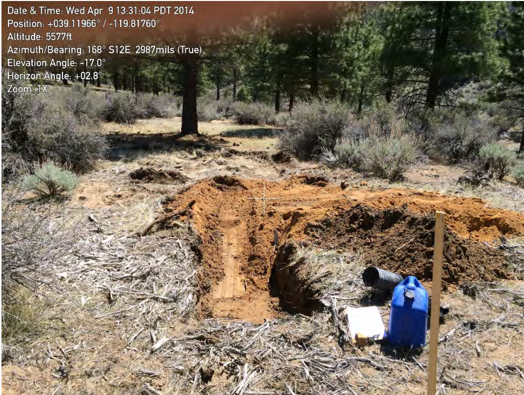
PHOTO 7 – Percolation Test Pit TP – 7.
