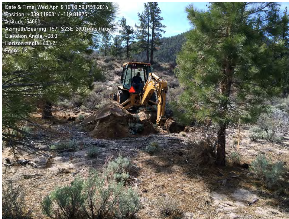
PHOTO 2 – Percolation Test Pit TP-2.
