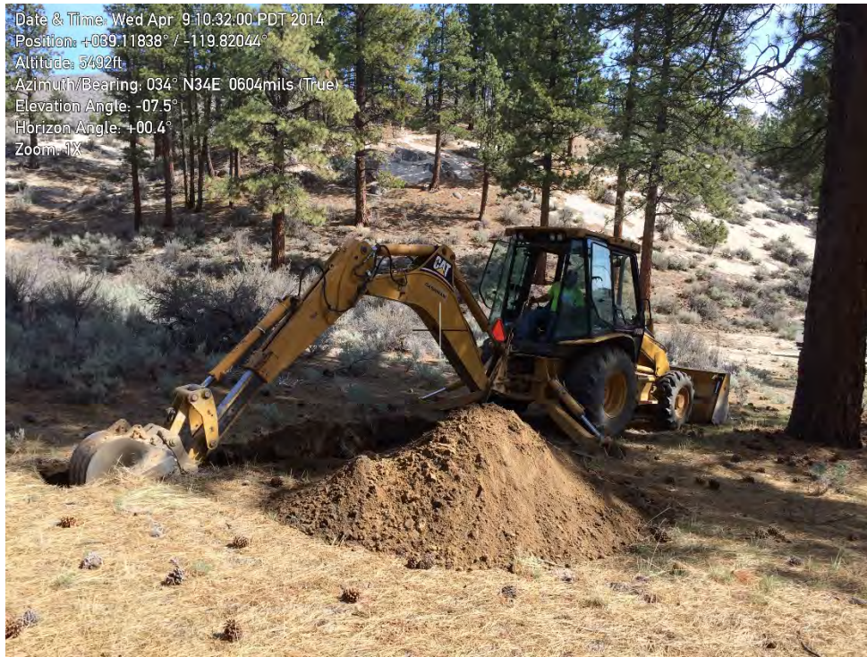
PHOTO 3 – Percolation Test Pit TP – 3.
