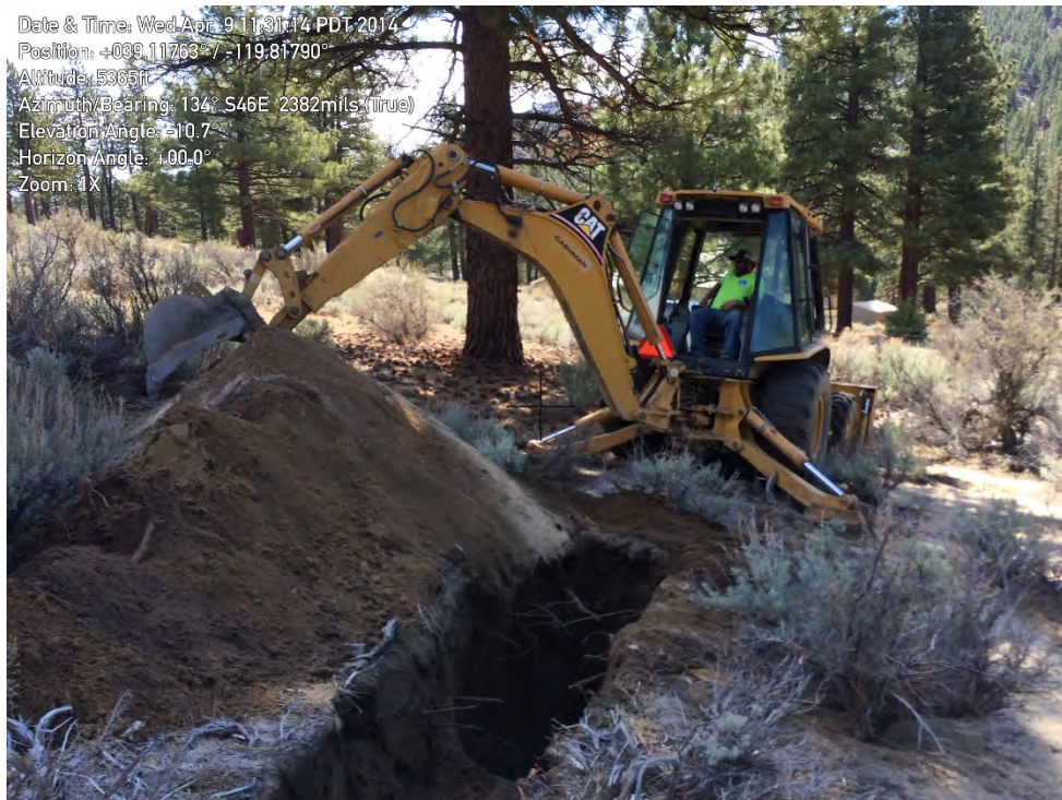
PHOTO 4 – Percolation Test Pit TP - 4
