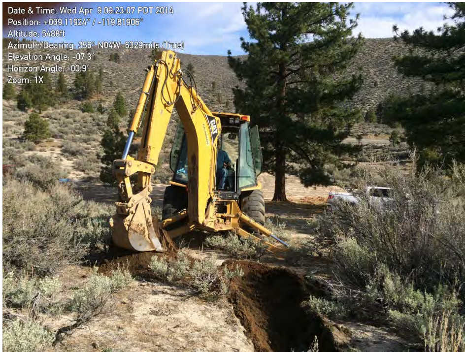
PHOTO 1 – Percolation Test Pit TP – 1.
