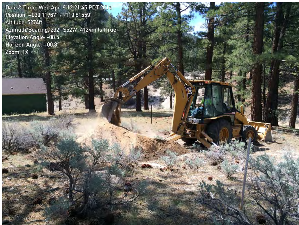
PHOTO 6 – Percolation Test Pit TP - 6
