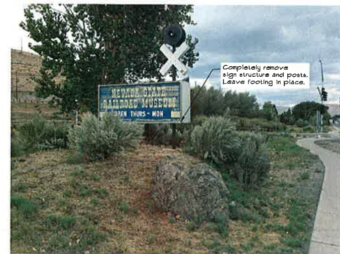
EXISTING SIGN TO BE REMOVED
