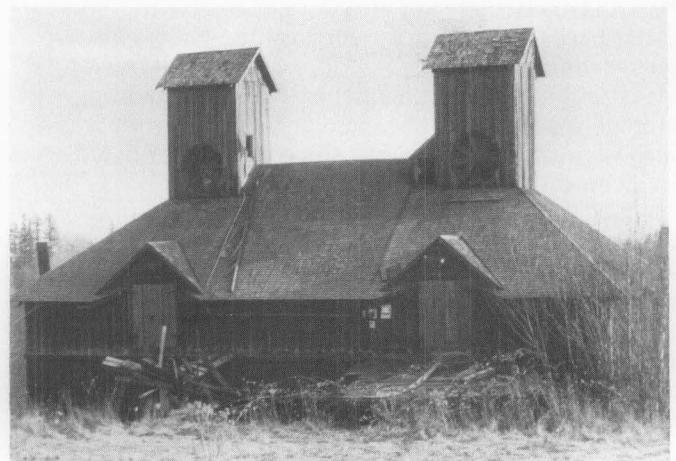
The two ventilating towers are the character-defining aspect of this Oregon hop-drying barn. Photo: Allan Nelson.
