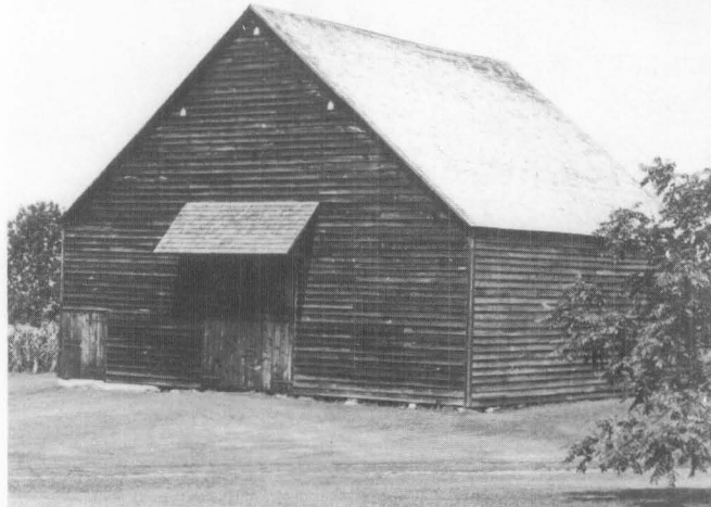
Built in the late 1700s, this New York Dutch barn survives in excellent condition. Gable roof, center wagon doors with pent roof, stock door at the corner and horizontal clapboarding are all typical features of the Dutch barn. Three holes for martins, traditional features of Dutch barns, can be seen near the top of the facade (they have been plugged and are lighter than the surrounding clapboards). Photo: Clarke Blair.
