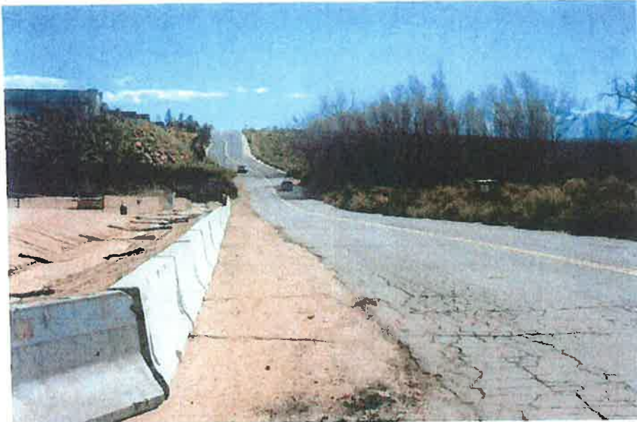
1 - Looking south on Vista Grande Blvd from Old Clear Creek Rd
