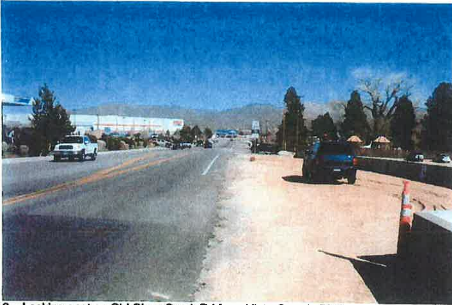
3 – Looking east on Old Clear Creek Rd from Vista Grande Blvd
