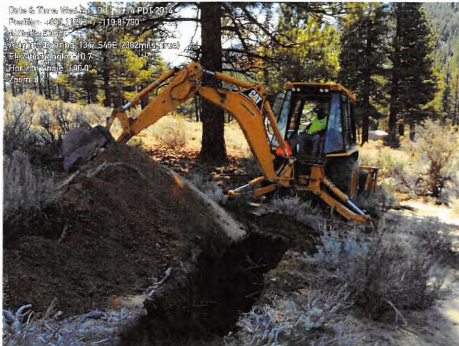
PHOTO 4 – Percolation Test Pit TP - 4
