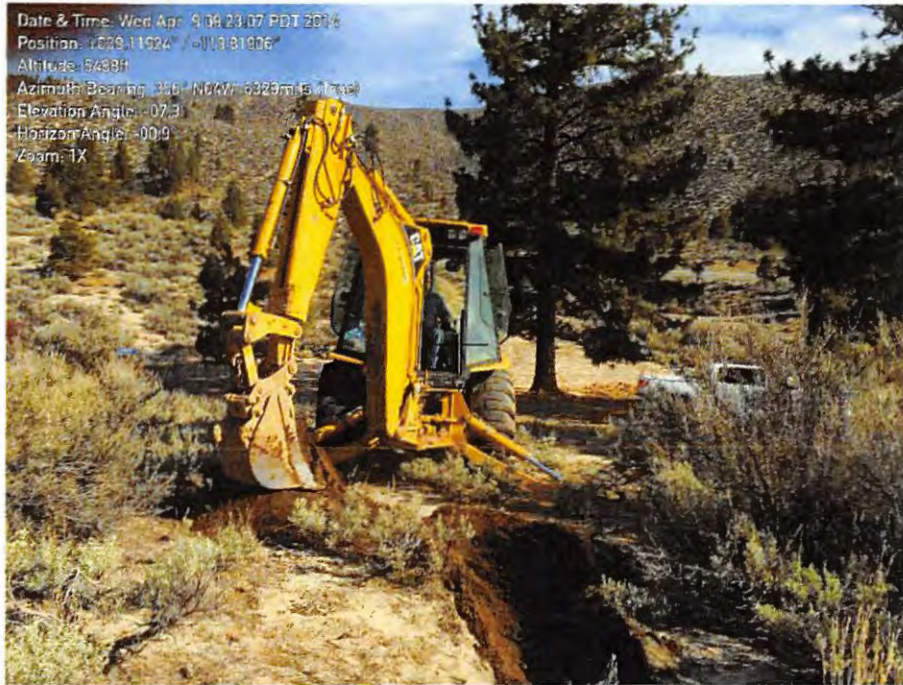
PHOTO 1 – Percolation Test Pit TP – 1.
