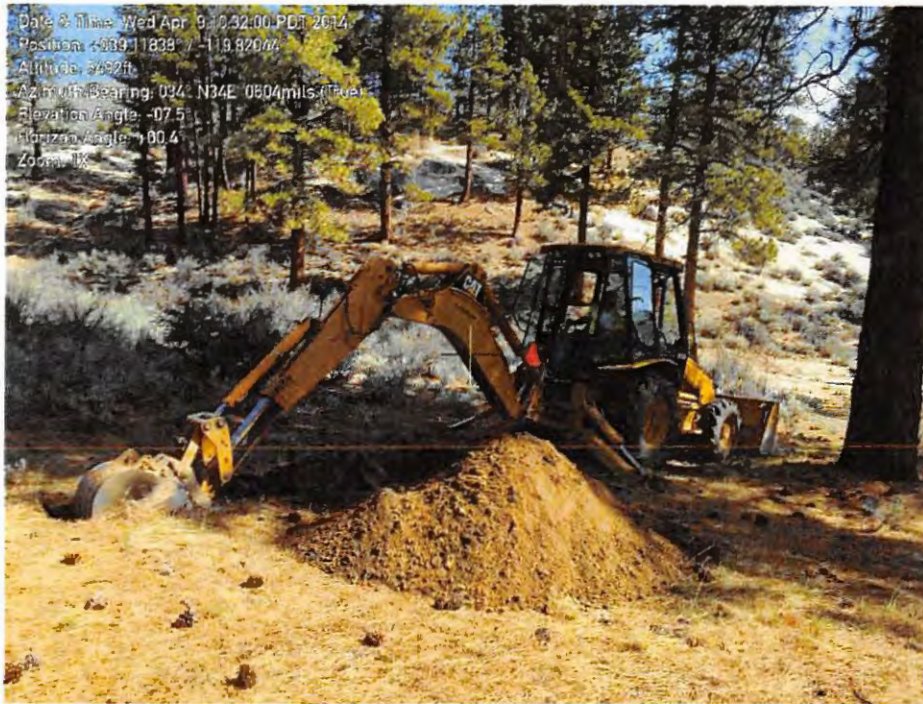
PHOTO 3 – Percolation Test Pit TP – 3.
