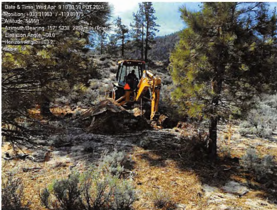
PHOTO 2 – Percolation Test Pit TP-2.
