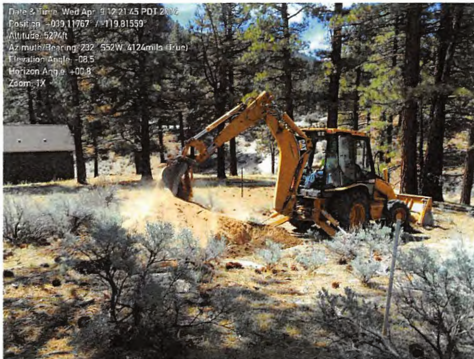
PHOTO 6 – Percolation Test Pit TP - 6
