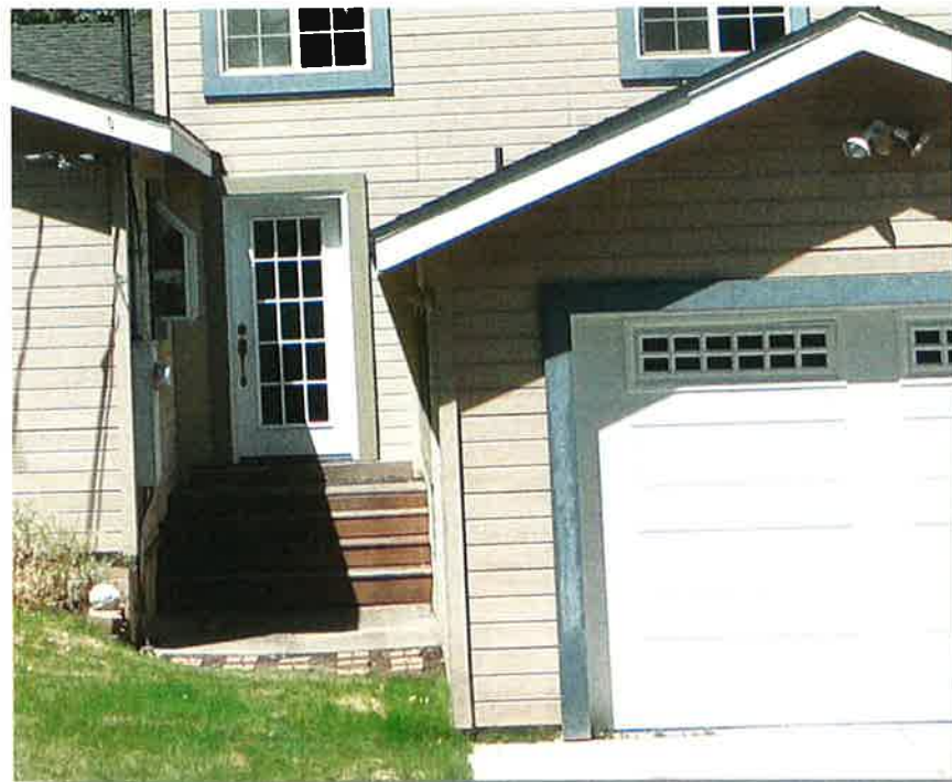
Figure 4. Close-up of existing West Elevation and the space to be occupied by the proposed pantry. Proposed pantry would occupy the space between the garage and the existing kitchen. The side entrance door and steps would be eliminated and electrical panel moved indoors.
