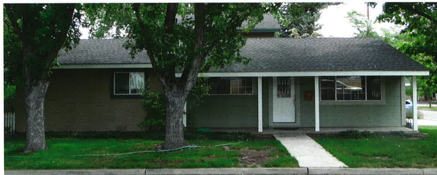
Figure 7. Existing west elevation view.
