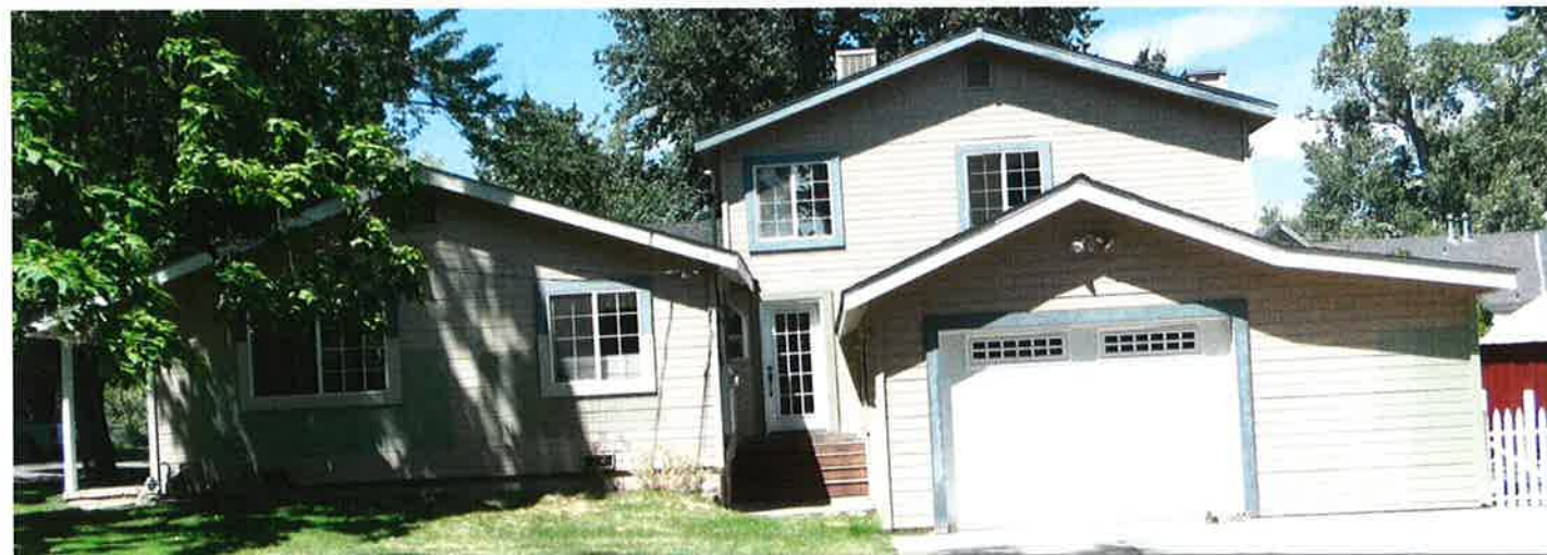
Figure 1. Existing south elevation view.
