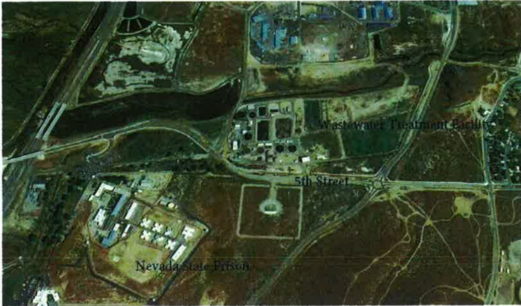
Aerial View of Wastewater Reclamation Facility (Google Earth)
