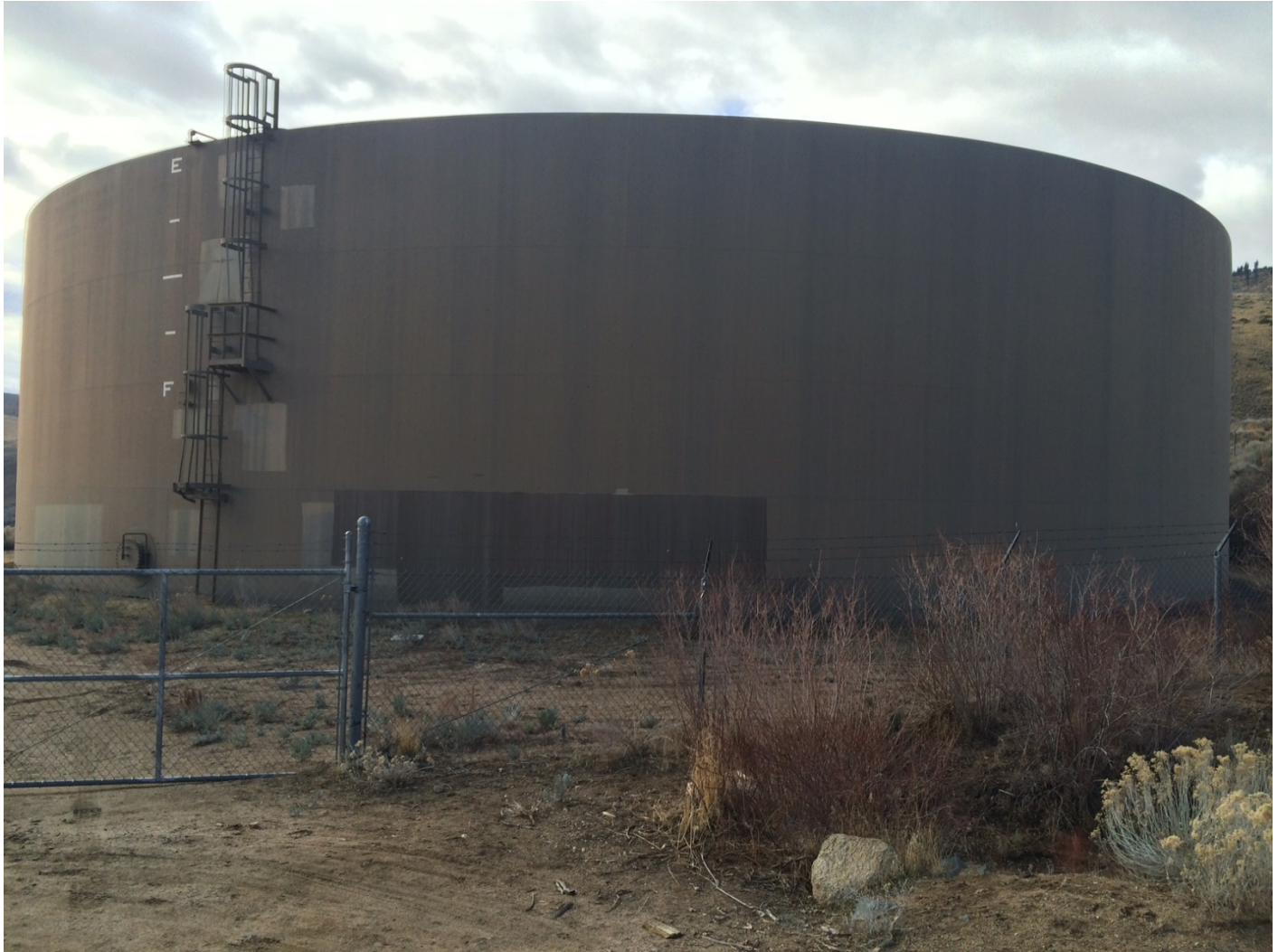
Photo 1: Ash Canyon Water Tank
