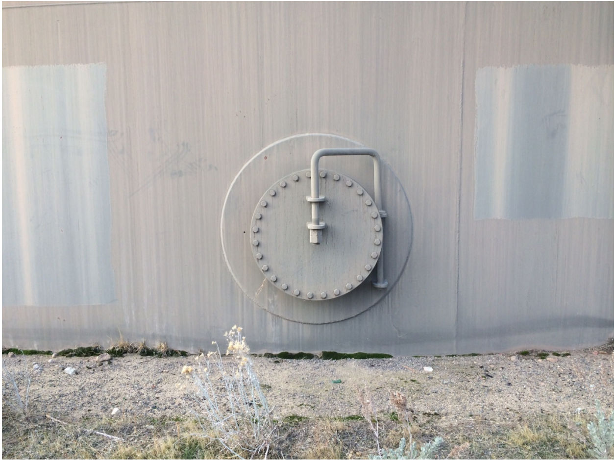
Photo 2: Ash Canyon Water Tank Access Manhole
