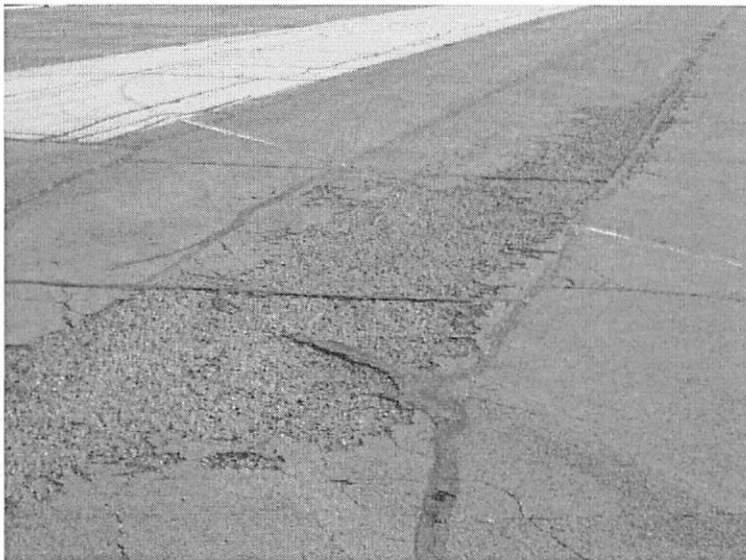
Typical raveling near the main taxiway in the north apron
