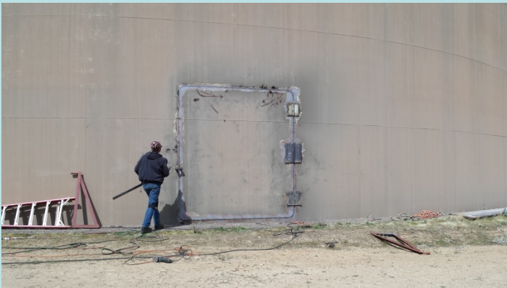
Ash Canyon Tank Rehab
